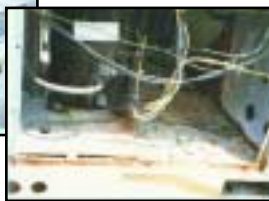
The air cavity of a unit with a rusted basepan
