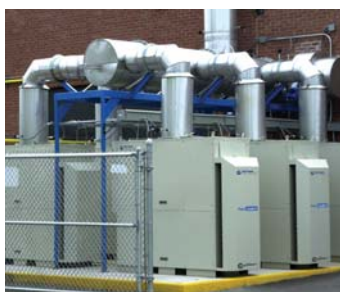
Microturbines (above) and the Absorption Chiller (below) are integrated to create the PureComfort™ 240M Solution
