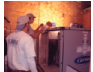
Installation of Carrier 39M Air Handling Unit
