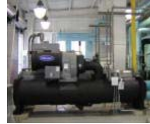
Installation of Carrier 19XRV 420 ton chiller
