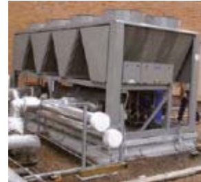
Installation of Carrier 30RB chiller
