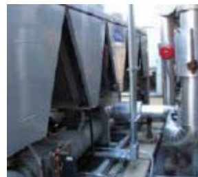
Installation of Carrier 30XA chiller
